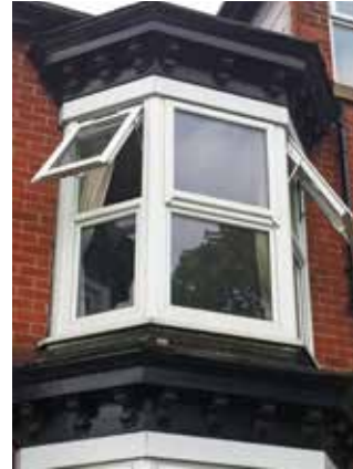
Mock sash bay window with top openers and tilt and turns below
