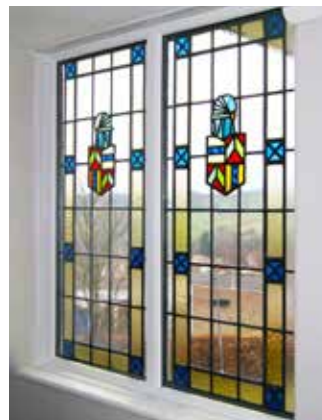
Window with original stained glass triple glazed
