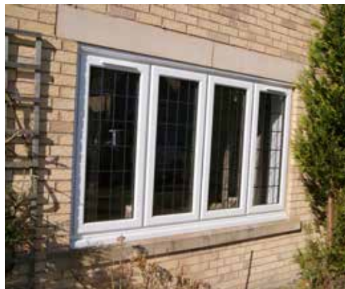
Casement window with lead, dummy sashes and side openers
