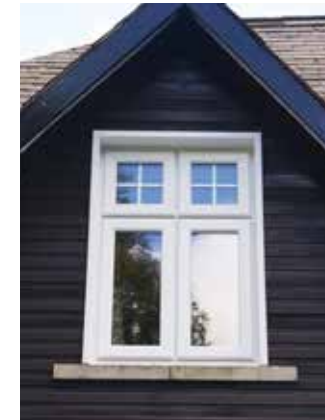
Casement window with dummy sashes and internal fret in top lights
