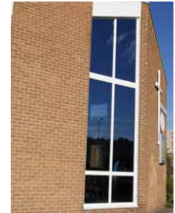
Large panoramic casement window with raked head
