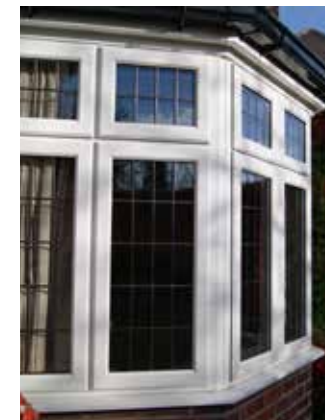
Bay with square lead and dummy sashes
