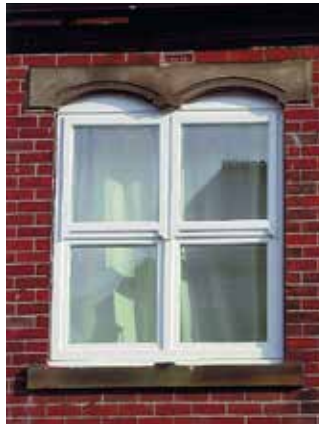
Mock sash window with top openers and tilt and turns below
